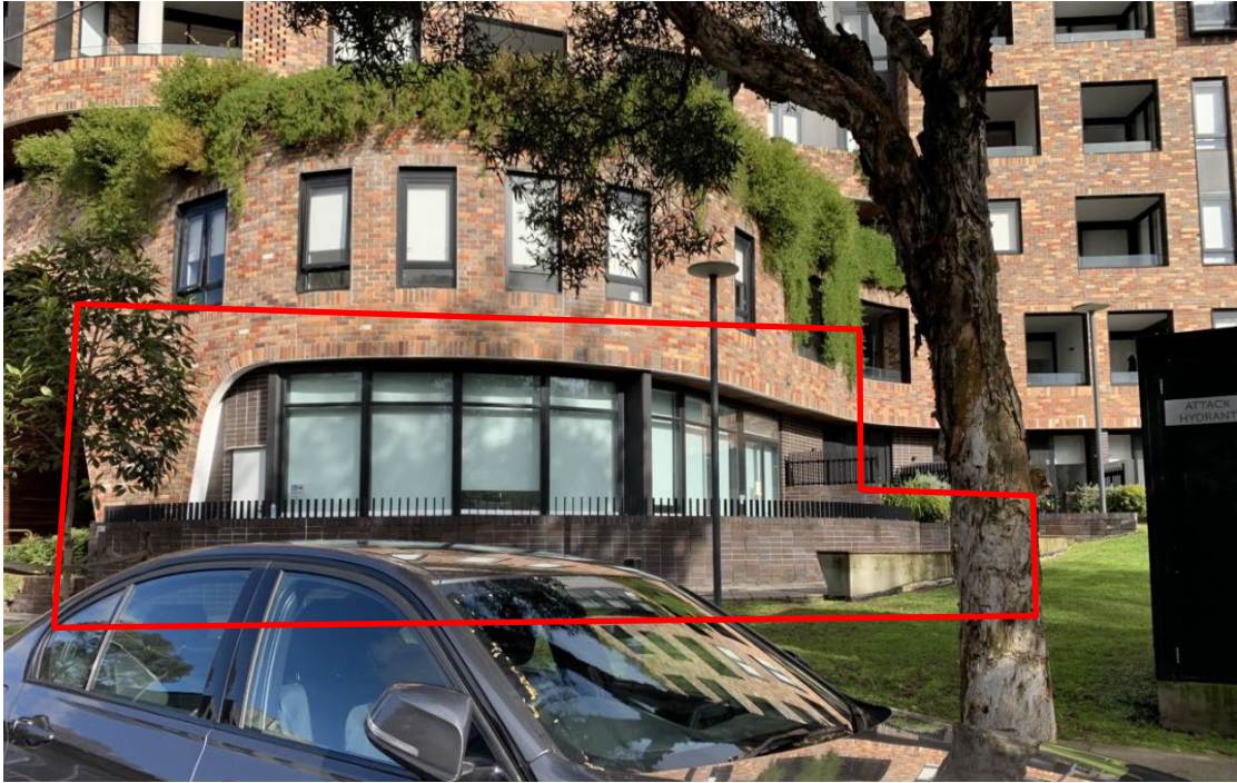
site as viewed from Huntley Street ground floor tenancy and outdoor terrace highlighted in red
